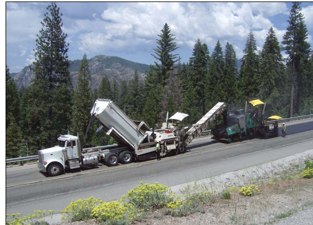
A truck feeds asphalt into machinery to apply a "bonded wearing course" on SR 20 east of Nevada City
