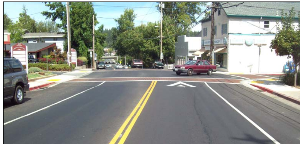
Major reconstruction on So. Auburn Street in Grass Valley was made possible with ARRA funding
