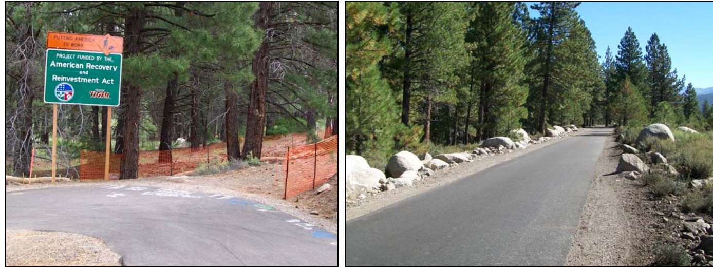
The Town of Truckee utilized $633,342 of ARRA funding to construct a segment of the Truckee River Legacy Trail pedestrian/bike path.
