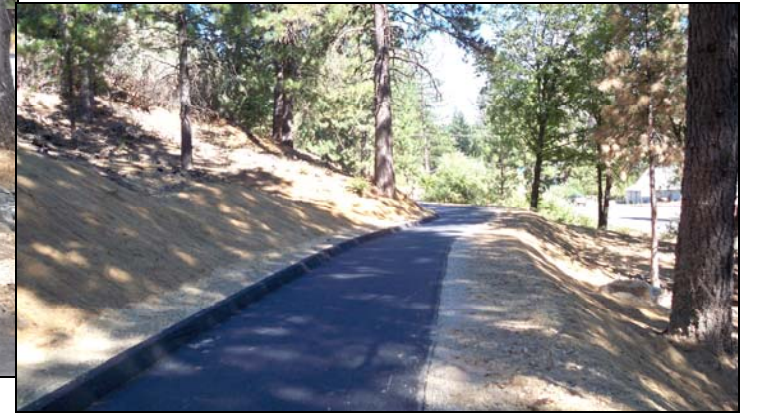
Pedestrian walkway from No. Bloomfield Rd. to Madelyn Helling Library at the Nevada County Government Center paid for with CMAQ funds
