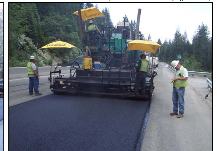
SR 20 surface overlay funded by Caltrans to address wear and tear on highway in 2009 from detoured traffic to accommodate I-80 construction
